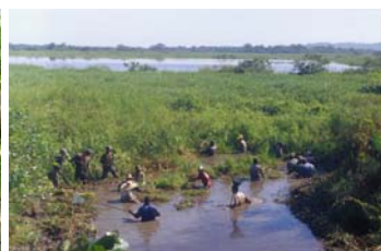
Hydraulic restoration of ciénaga Las Flores
